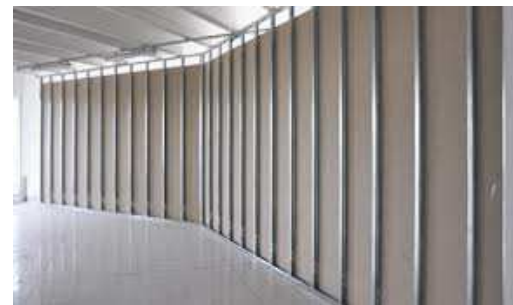
Internal structure of a plasterboard wall
