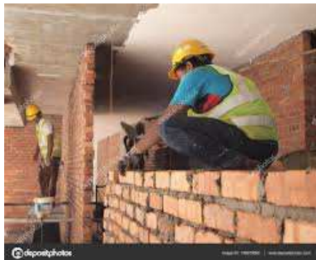
BRICKS (usually covered with a layer of plaster and another layer of painting)
